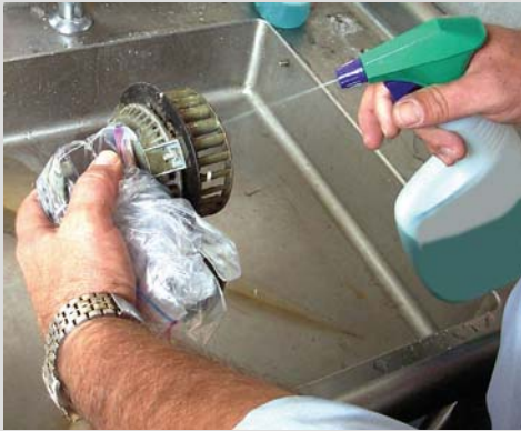
Cleaning the blower motor ensures even combustion.
